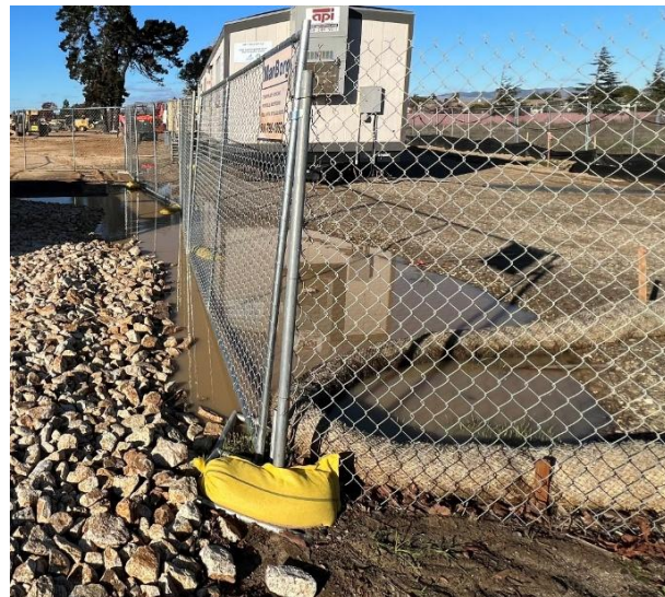
Prevent runoff from construction activity
