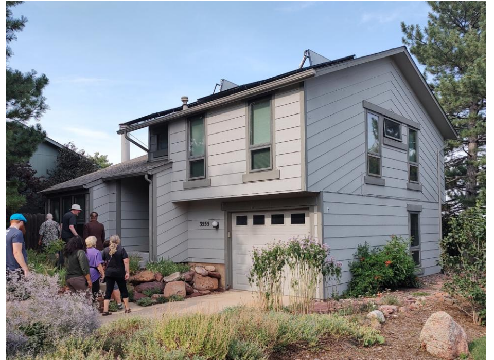
ASES Solar Homes Tour 2025 –Existing Home retrofit for ZNE includes triple paned windows.
