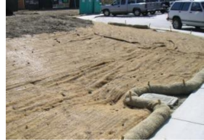
Burlap mat & straw wattles at catch basin
