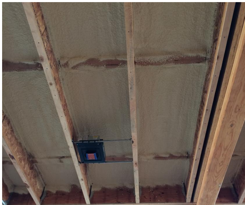
2" Closed Cell Spray Foam is adhered to underside of roof deck.
