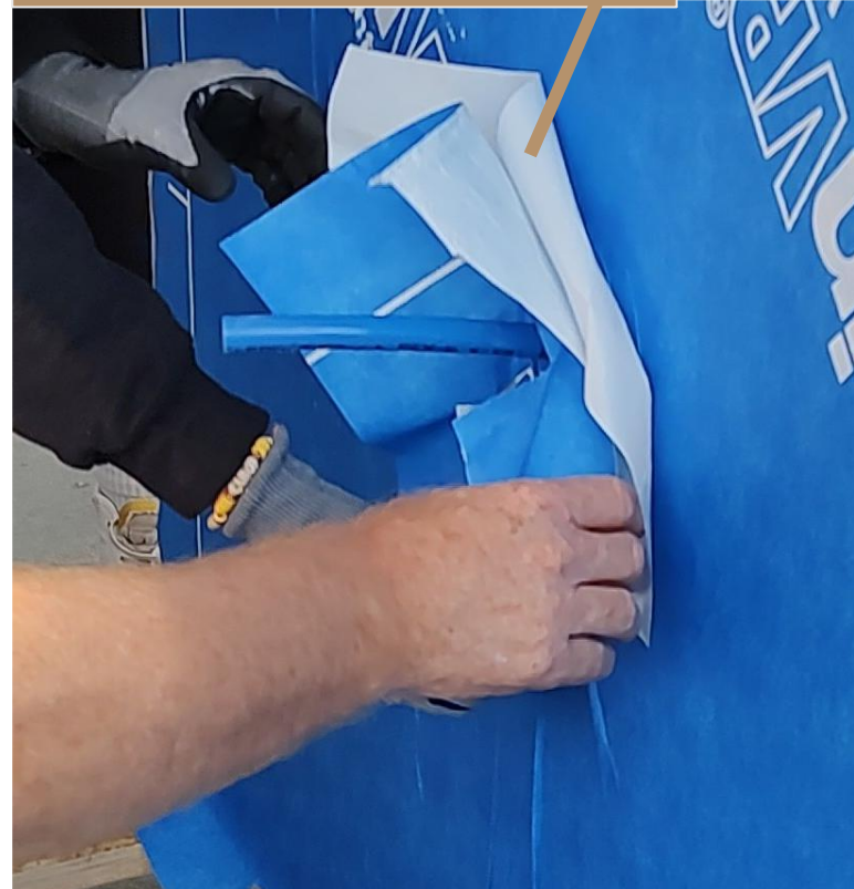
Taped and Sealed – Using Pieces of the Self-Adhered Membrane
