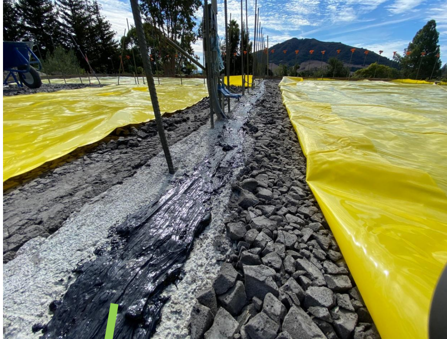
Mastic is brush applied to concrete footing or grade beam
