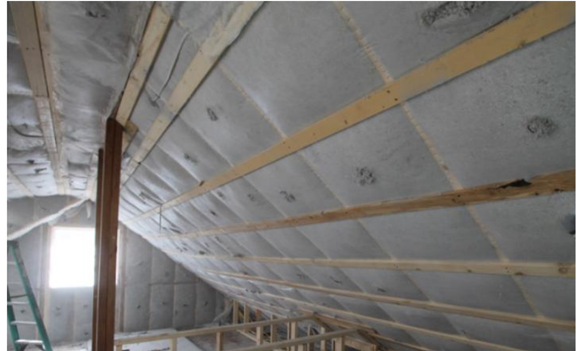
Blown-in Insulation at Underside of Roof/Ceiling
