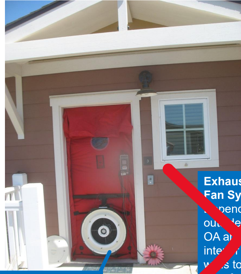
Blower Door Compartmentalization Testing
