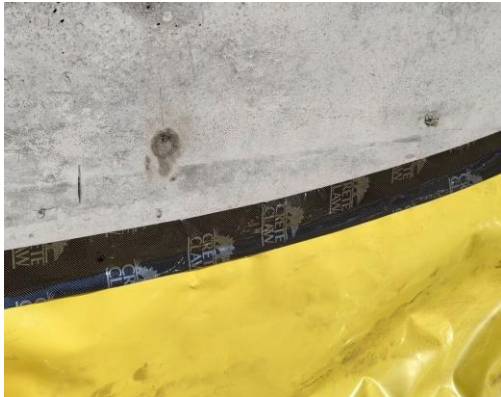
Use specialized tape and/or mechanical fasteners – typically sold with the vapor barrier -- securely attached to the foundation
