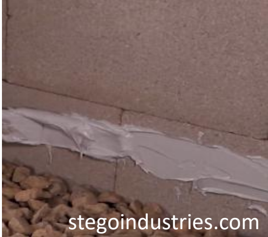
Use specialized tape and/or mechanical fasteners – typically sold with the vapor barrier -- securely attached to the foundation
