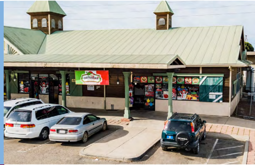
Incentives for Tortilleria Mexico #4 in Santa Maria supported a heat pump water heater project.
