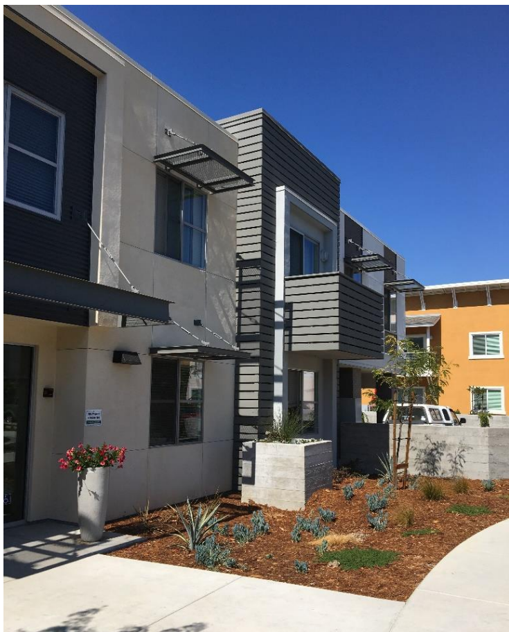
860 on the Wye – Multi-Family Low-Rise All-Electric Zero Net Energy
