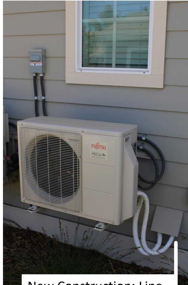
New Construction: Line Set Built-In to Wall
