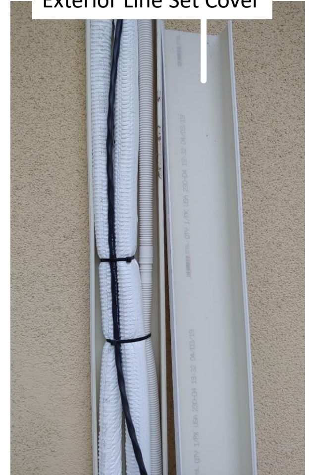
Remodel: Exterior Line Set Cover
