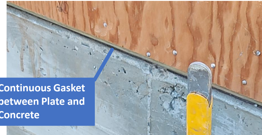
Exterior Bottom (Sill) Plates Sealed to Floor
