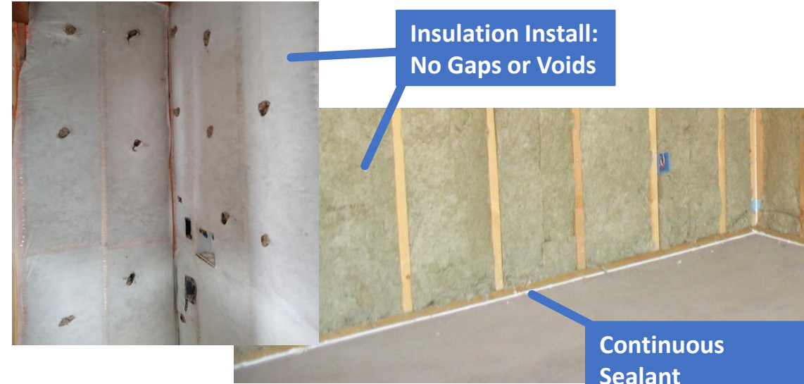
Exterior Bottom (Sill) Plates Sealed to Floor
