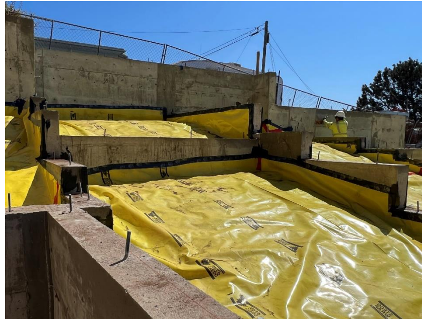
Vapor retarder installed over gravel for capillary break
