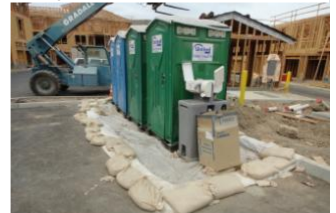
Prevent runoff from construction activity
