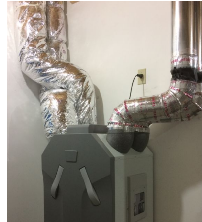
Intake and exhaust duct insulation
