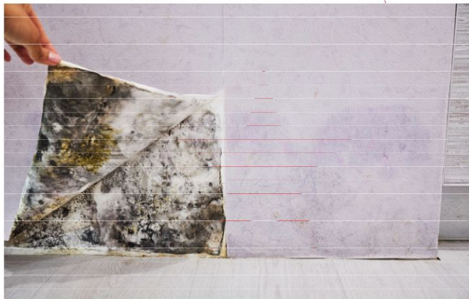
Vinyl Wallcovering – Mold due to inwardly driven moisture trapped by the vapor impermeability of the vinyl wallcovering
