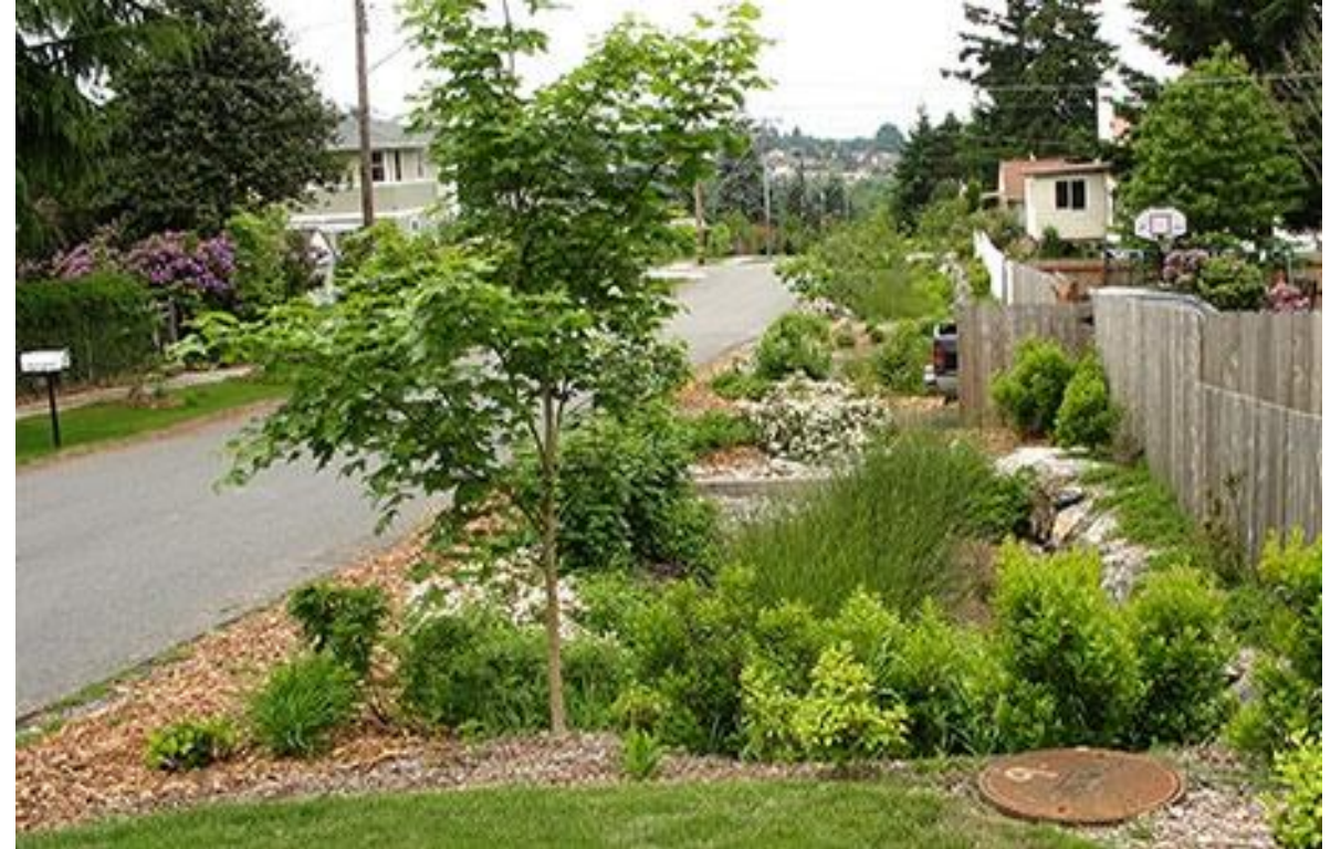
South Thornton Natural Drainage System ( NDS ) Project, Seattle, WA Permeability to slow, spread and sink rainwater
