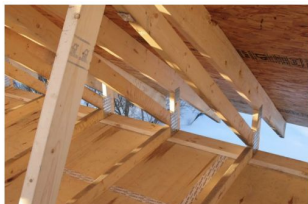
Photo of roof plywood air tight layer seams taped, roof trusses before insulation install.
