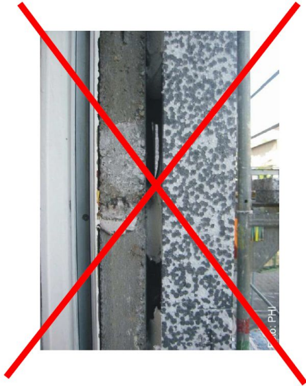
Gap filled with adhesive
