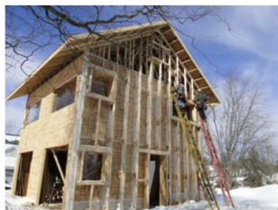
Photo of remote wall wood truss installed on east wall with poly film air tight layer lapped up wall OSB sheathing.
