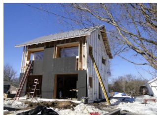
Photo of weather barrier on east wall with rainscreen battens, fiberboard sheathing on south wall.
