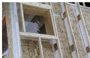
Photo of OSB air tight layer seams taped, plywood window box, and remote wall truss.
