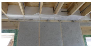
Photo of dense packed cellulose installed in 2x4 stud wall and insulation between floor joists.
