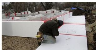
Photo of EPS foam around concrete slab-on-grade, EPS frost skirt, and poly film air tight layer.
