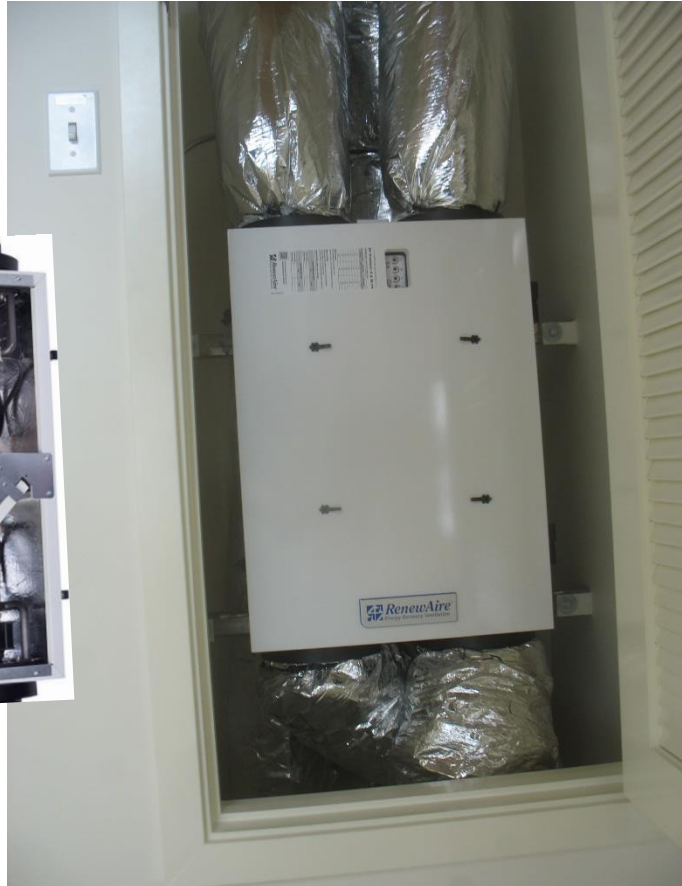
Balanced Ventilation ERV Provides Outside Air (OA)
