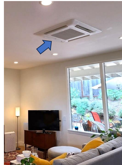
Ductless Recessed-Ceiling
