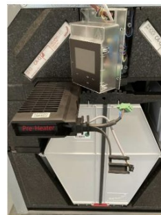
HRV built-in pre-heater unit
