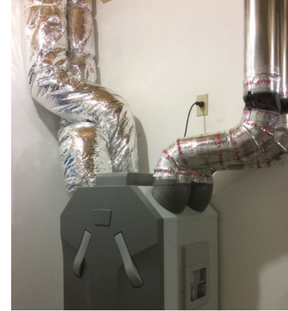
Intake and exhaust duct insulation
