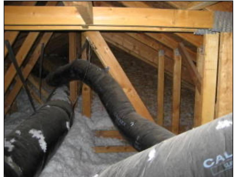
These ducts are above the insulation
