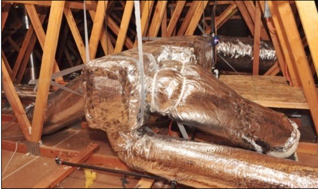
These ducts will be buried in insulation
