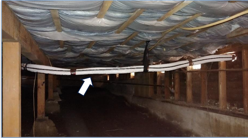
Refrigerant and Communication Line Set – Raised Floor
