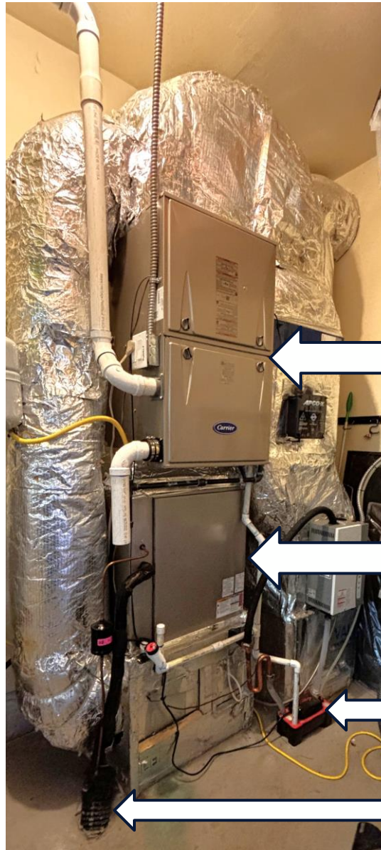
New Higher Efficiency Furnace
