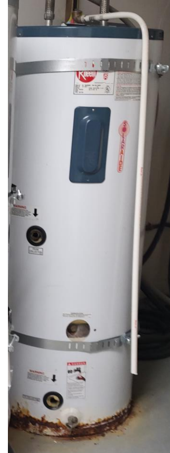
Electric Tank – Leaking at base
