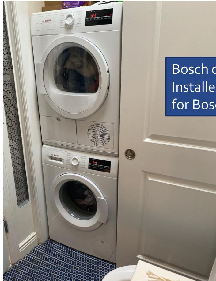
Closet: Stacked Washer with Heat Pump Dryer
