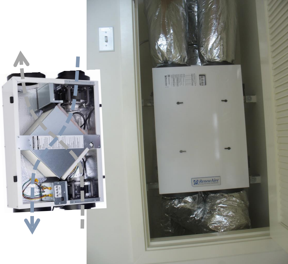
Balanced Ventilation ERV Provides Outside Air (OA)
