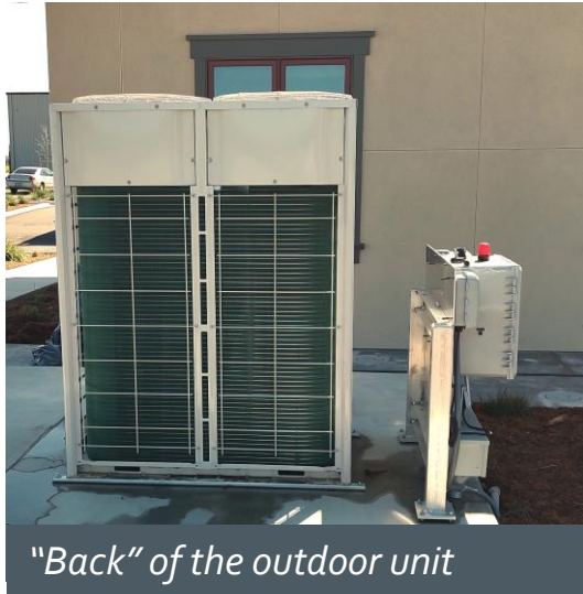
Winery Laboratory and Office – multi-zone VRF with ducted fan coil units
