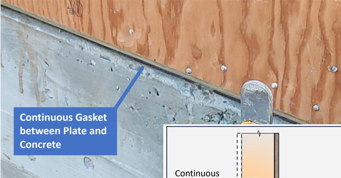
Continuous Gasket between Plate and Concrete
