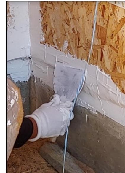
Structural sheathing is ready for a liquid applied membrane, self-adhered membrane, or drainage plane stucco wrap.
