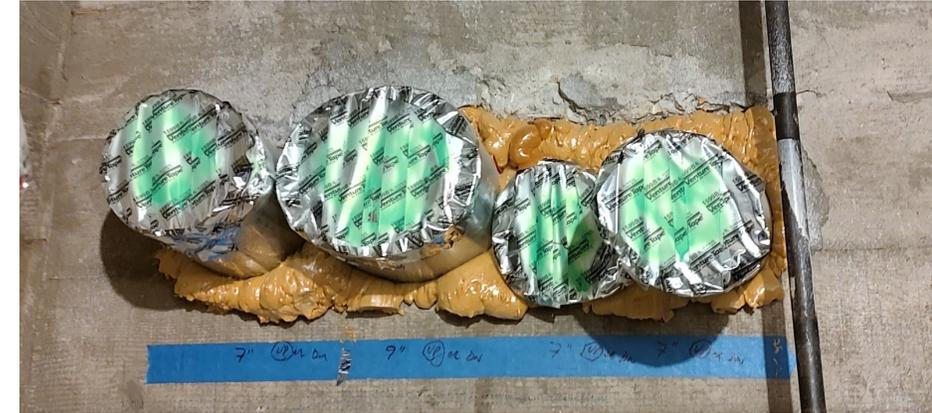
Conditioned 'Daylit' Basement to Crawl Space – Penetrations are air sealed and walls will be insulated.
