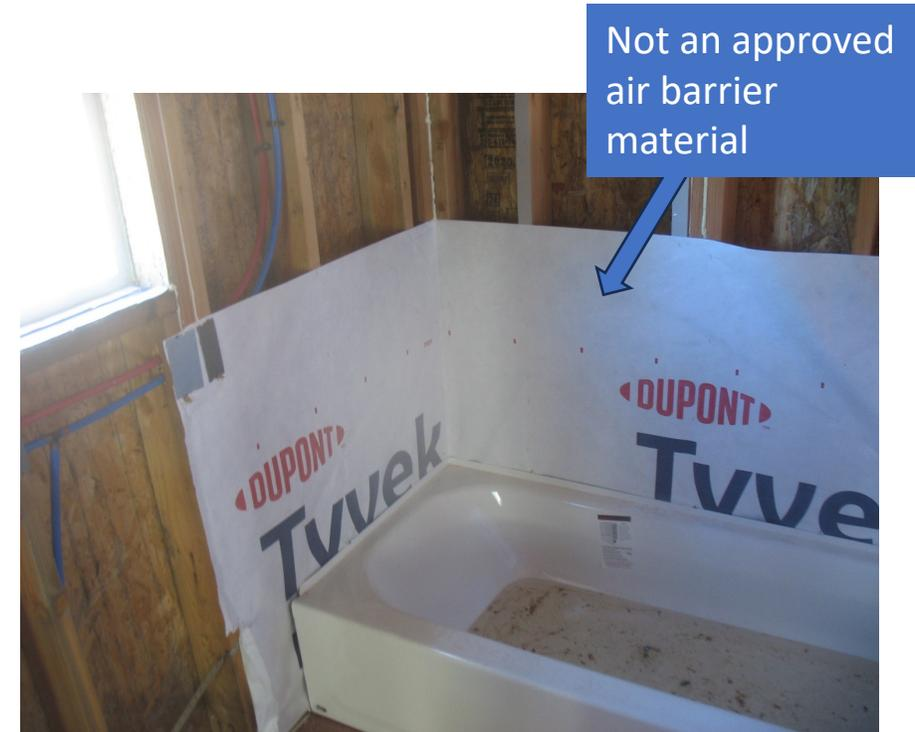
Proper insulation and air-barrier missing behind tub at the exterior walls.
