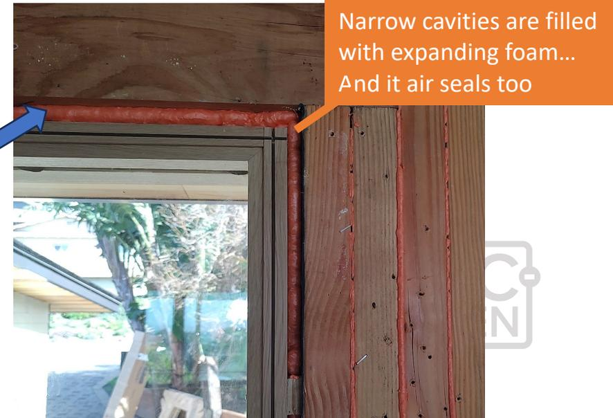
Narrow cavities are filled with expanding foam... And it air seals too
