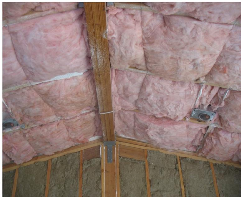
Remaining cavity is filled with Batt Insulation. (Blown-in insulation would also be acceptable.)
