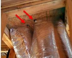
SPF can serve as a draft stop as long as it meets the minimum thickness required to be an air barrier.
